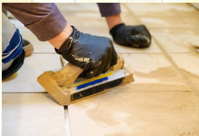
Application of Grout Admixture with H.P Grout in Grout Joints
