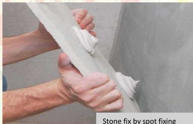
Stone fix by spot fixing
